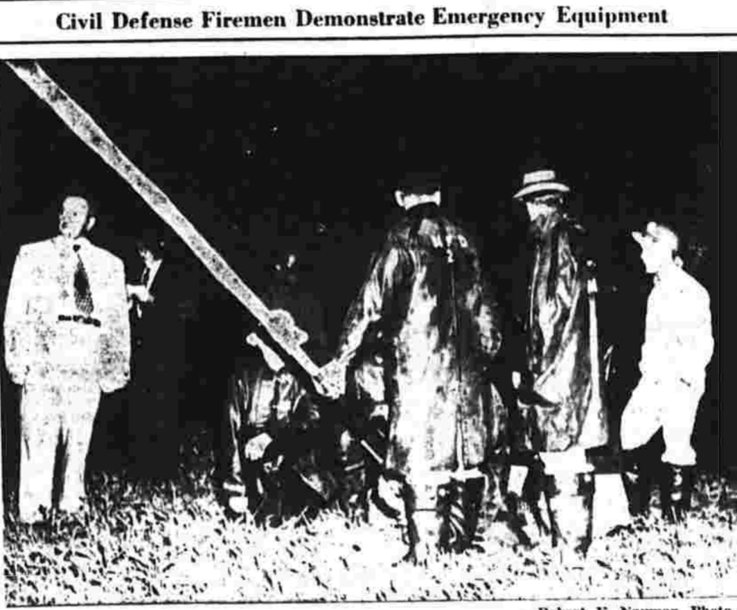
Civil Defense firemen last night laid 1,000 feet of four-inch pipe to test it worked. That water is coming out of that nozzle at about 540 gallons per minute, which is pretty good for an emergency pipe. The display was one phase of a demonstration for about 30 CD directors from the Hartford area. The CD heads were here last night as guests of Chief of Police Herman O. Schendel, local director, who showed them the progress Manchester has made in civilian defense.
